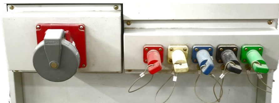
Figure 2.6 - Additional Power Supply
